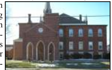
Elevator addition, Gothic arches
