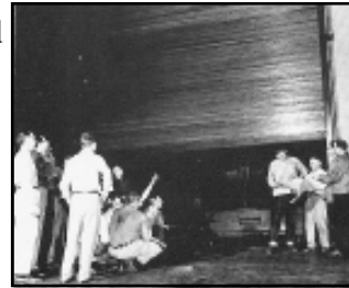
"Roll-top" divider between the Sunday School auditorium and the back of the sanctuary
